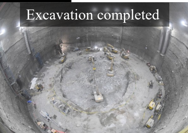
The largest man-made cavern in the world
